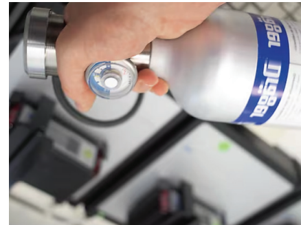
Check for leaks in the gas supply.
