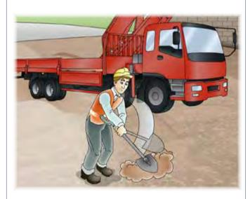
Check that the crane can be set up level. Don't use the crane unless it is level. Also check that the boom can move through its full range of movement without hitting overhead electric power lines or other obstacles.
