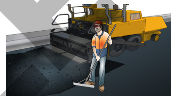
1. Stand at edge of asphalt area
