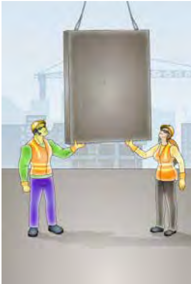
Preparing to move a concrete slab into place
