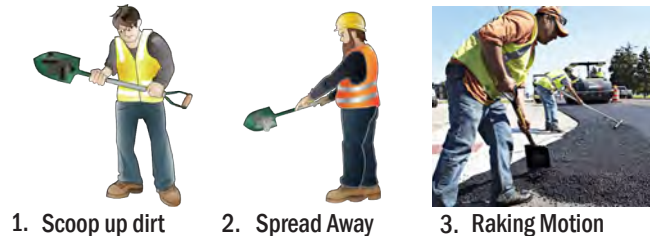
Hand spreading asphalt using a shovel
