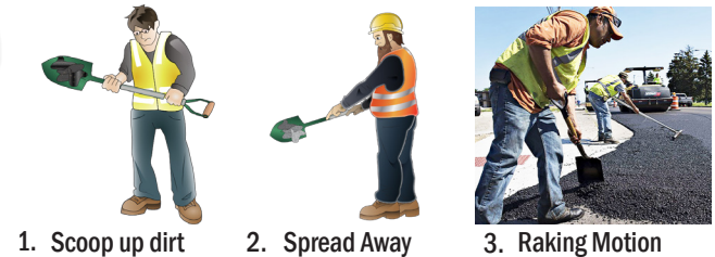
Hand spreading asphalt using a shovel
