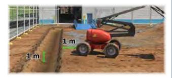
You should allow extra distance if the ground is soft or recently backfilled.
