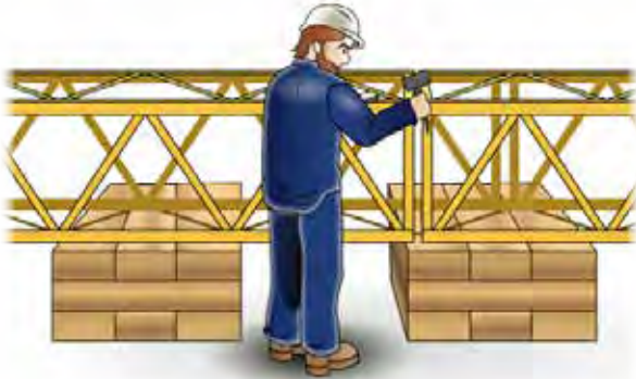
Dismantling of cranes on site
